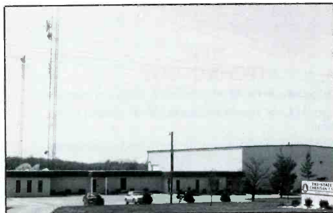
A view of the WTCT facilities, from the outside.
