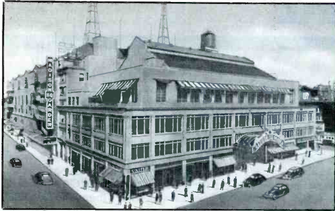
New York City's second Madison Square Garden once housed a radio station with the call letters WMSG. Note the towers on the roof.
